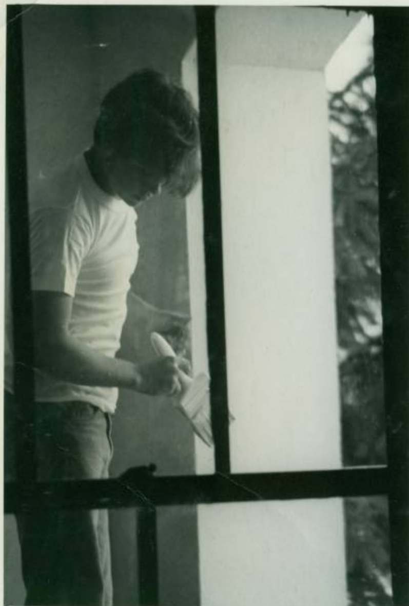
Kim Atha painting the windows - not the frames, the windows!
