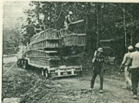
Unloading trusses for the new house.
